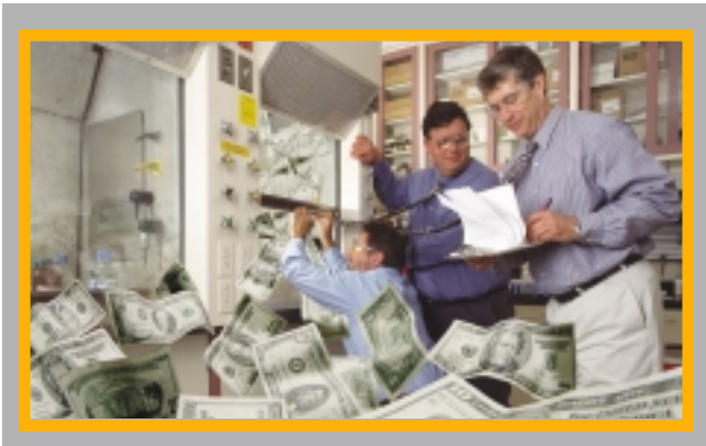
From left, Doug Christie, refrigeration mechanic, Rahway; Keith Williams, process manager, Stonewall; and Vincent Gates, department head, Rahway Power Plant, track down one culprit of energy loss at Merck -- open laboratory fume hoods.
